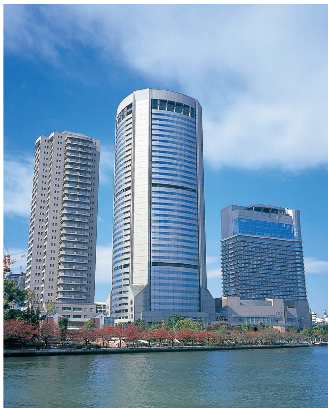
OAP Towers 帝国ホテル棟 (MSシール)
